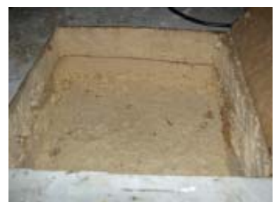
Core Sampling a 'dry' panel
