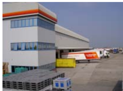
Phase IV Building
