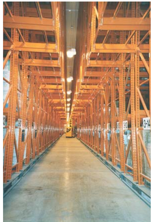
Typical Mobile Racked Store
