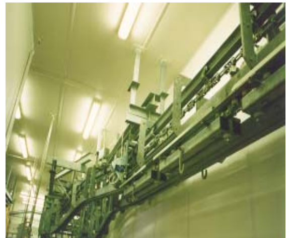
False Insulation Ceiling
